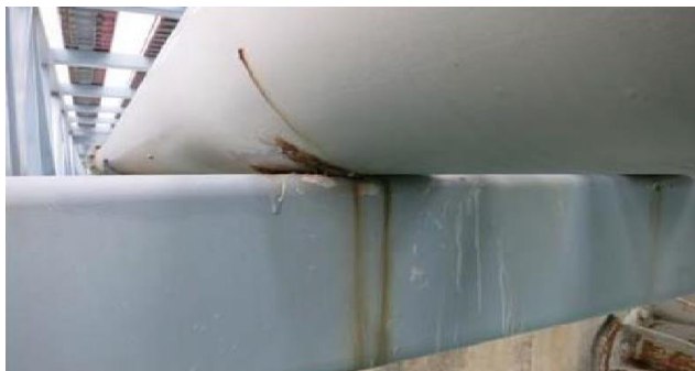
Unprotected Pipe
