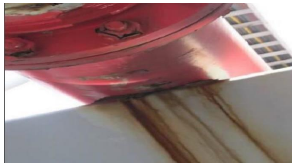
Corroded Pipe
